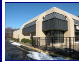
94 Car Parking Lot
